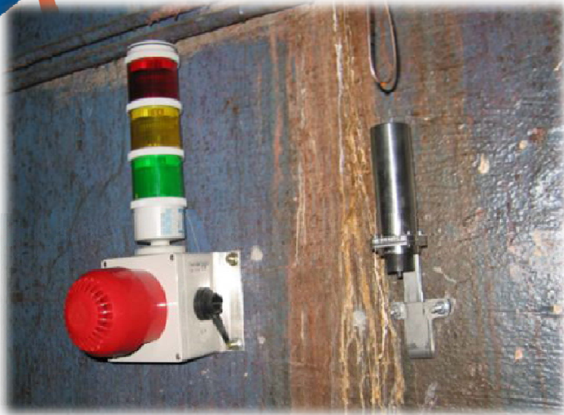
SRMS - GDR (gamma) sensor and sound and light signal device
