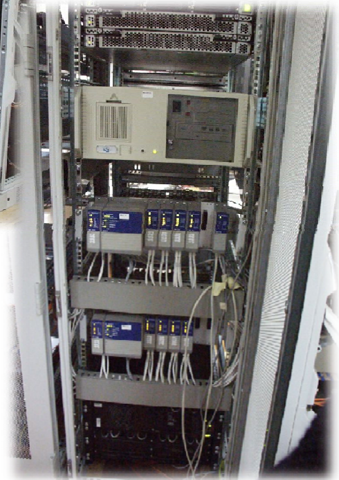
IMS-DCUs cabinets, installed in ChNPP room G-305
